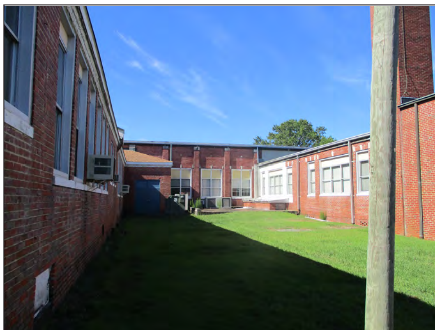
Photograph 10: View of the 1933 library addition; looking south. (2018)
