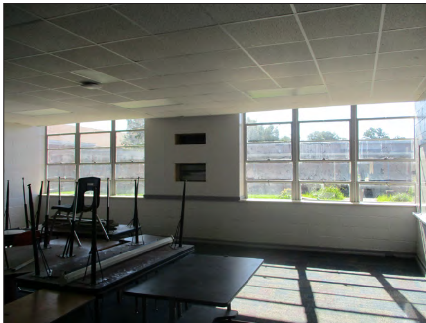
Photograph 26: Interior of 1953 classroom addition; looking east. (2018)
