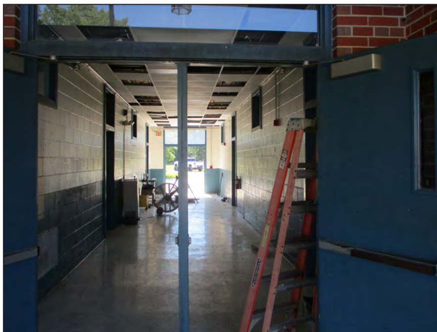
Photograph 30: Interior view of Annex; looking east. (2018)
