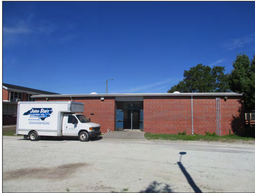
Photograph 29: View of Annex's east elevation; looking west. (2018)
