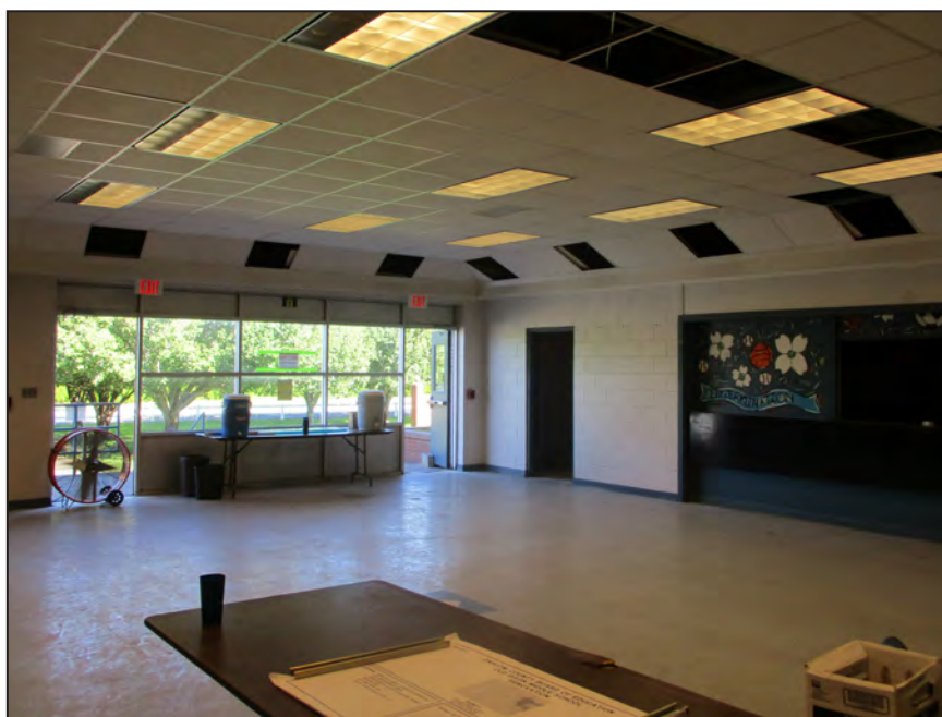
Photograph 27: Interior view of gymnasium lobby; looking northwest. (2018)
