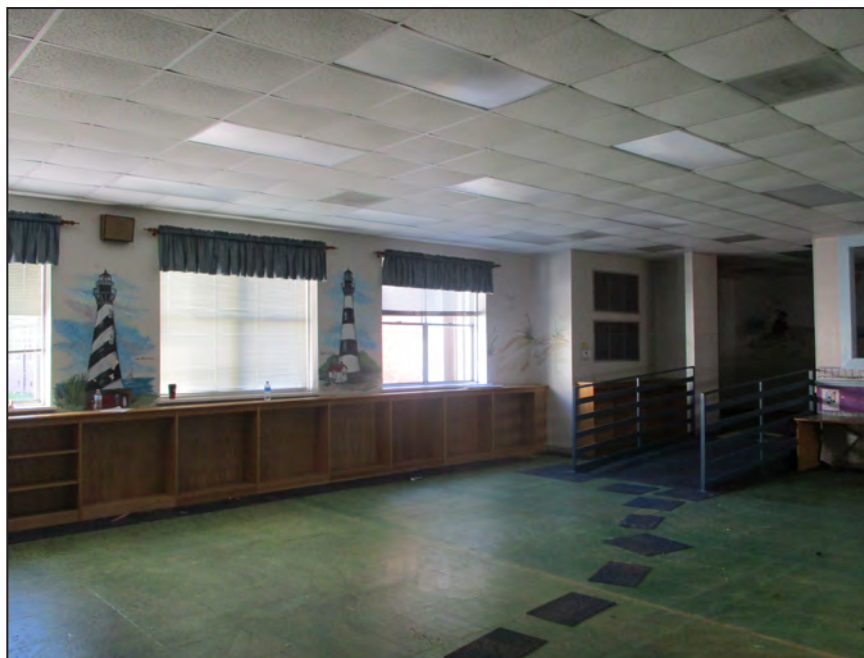
Photograph 11: Interior view of library addition; looking northeast. (2018)
