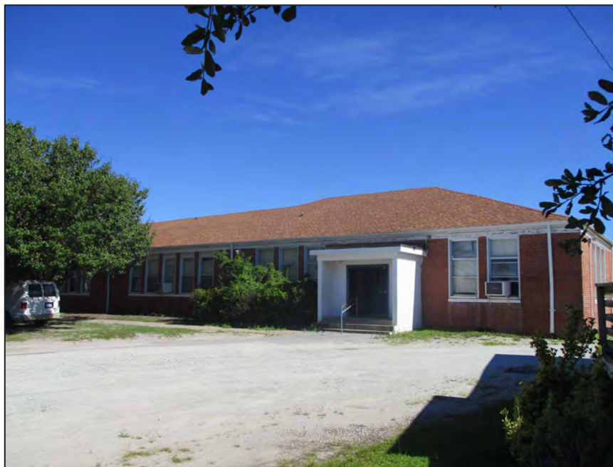
Photograph 15: View of Back Hall's south wing; looking north-northwest. (2018)
