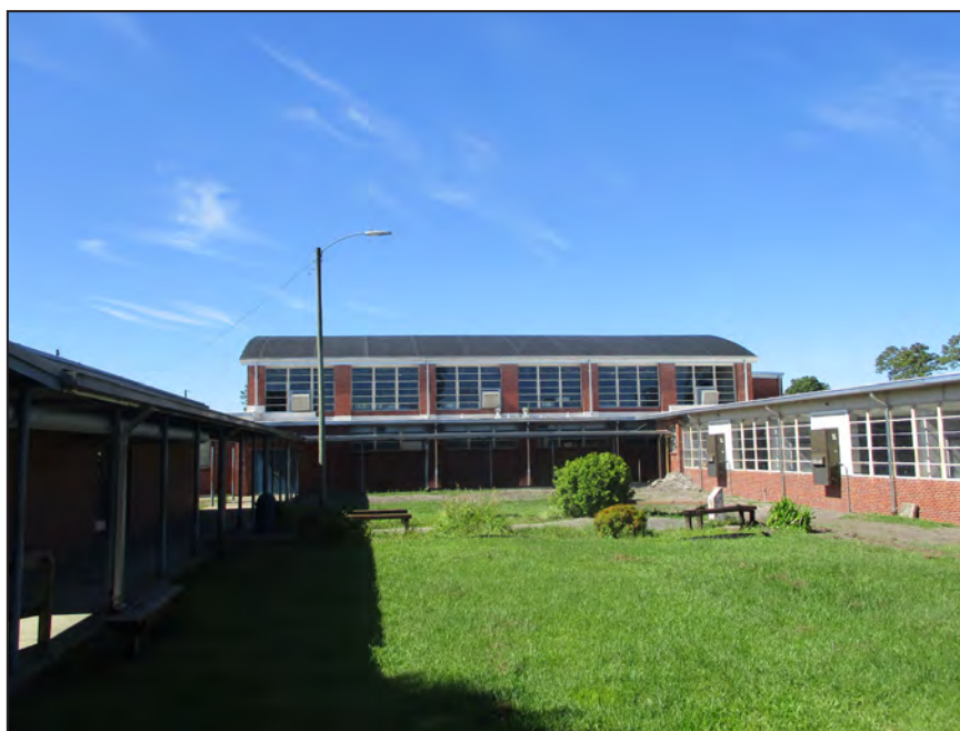
Photograph 25: View of gymnasium and north wing; looking south. (2018)
