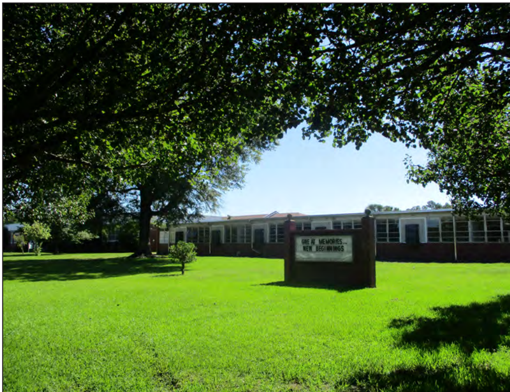
Photograph 21: View of west elevation of 1953 classroom addition; looking east-northeast. (2018)
