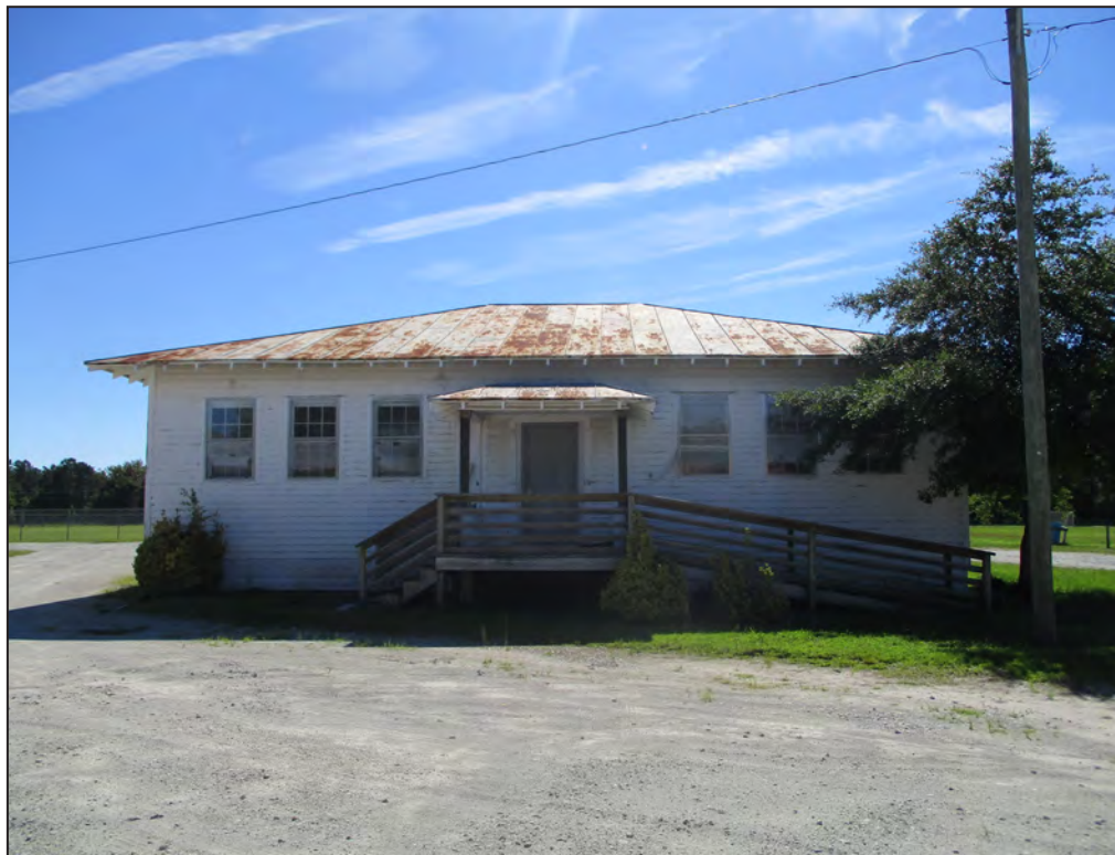
Photograph 31: View of original gymnasium (ca. 1927 frame building); looking east. (2018)
