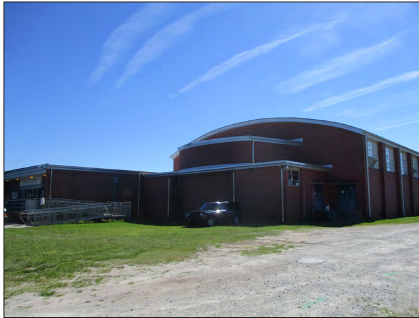
Photograph 22: View of gymnasium lobby and west wing; looking northeast. (2018)
