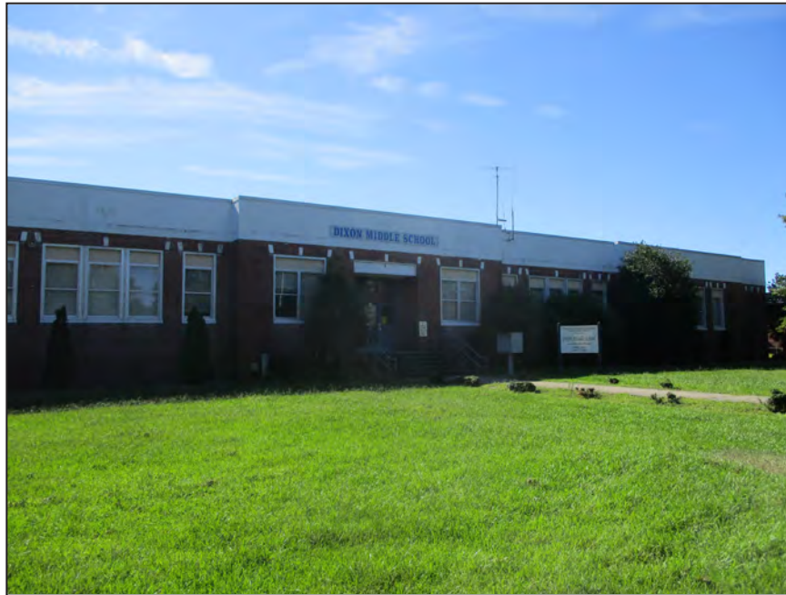
Photograph 5: View of Front Hall façade; looking east. (2018)
