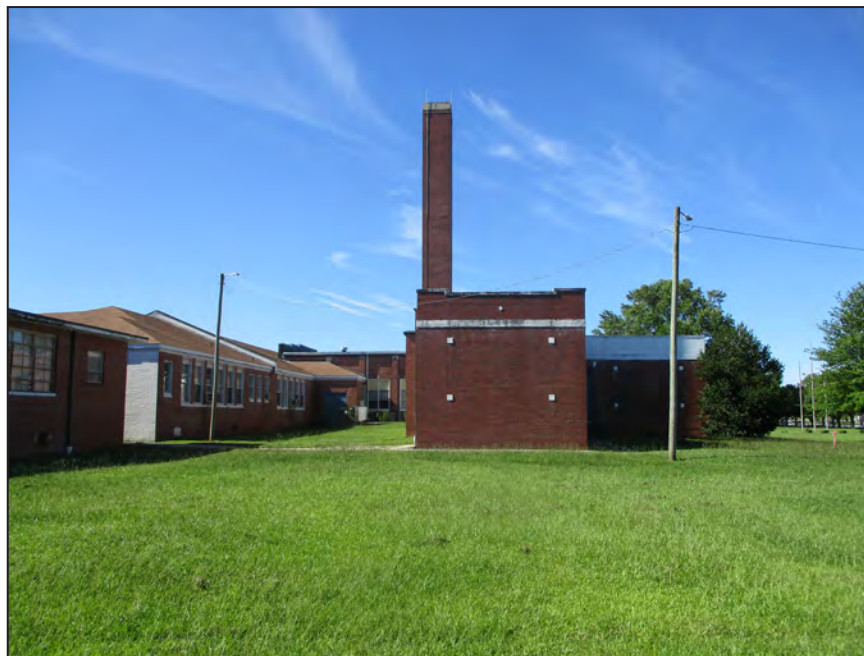
Photograph 6: View of Front Hall and boiler room's north elevation; looking south. (2018)
