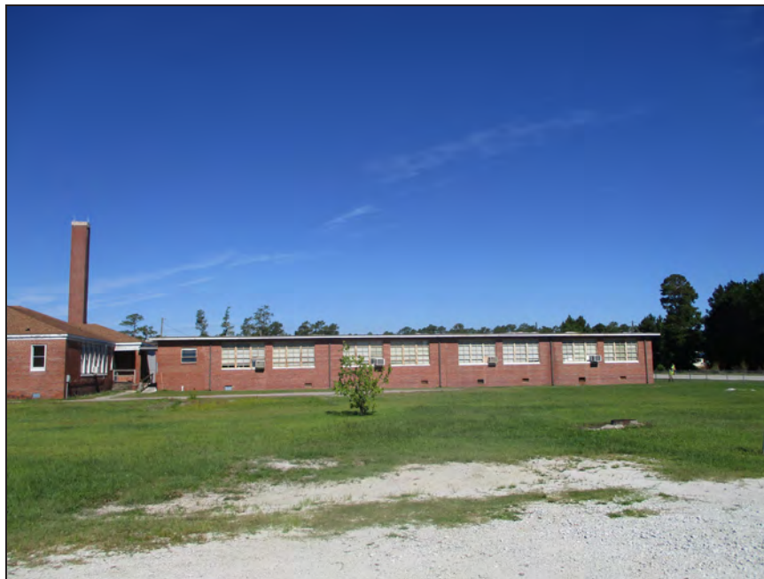
Photograph 19: View of wing addition (ca. 1945-1956); looking west. (2018)
