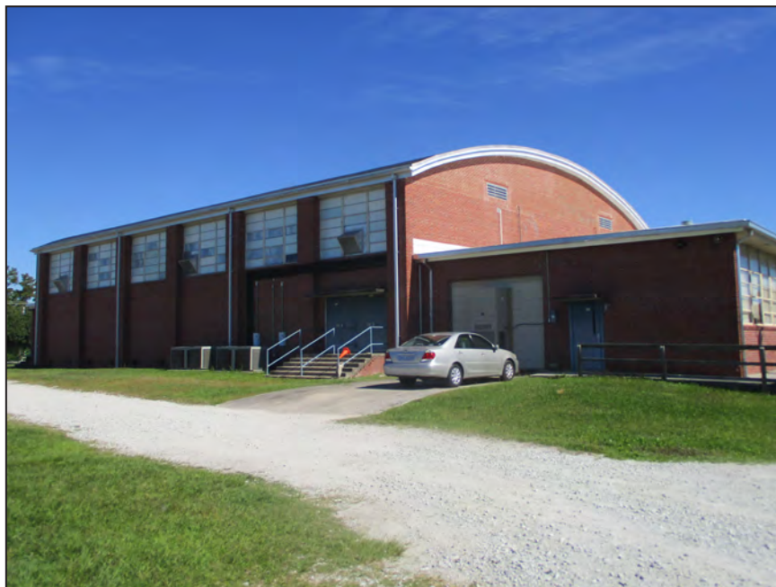
Photograph 23: View of gymnasium and band room's south elevation; looking northwest. (2018)
